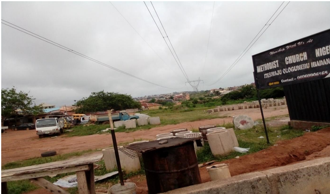
Figure 4.4 Buildings and Business Activities Under 33kva High Tension Wire
