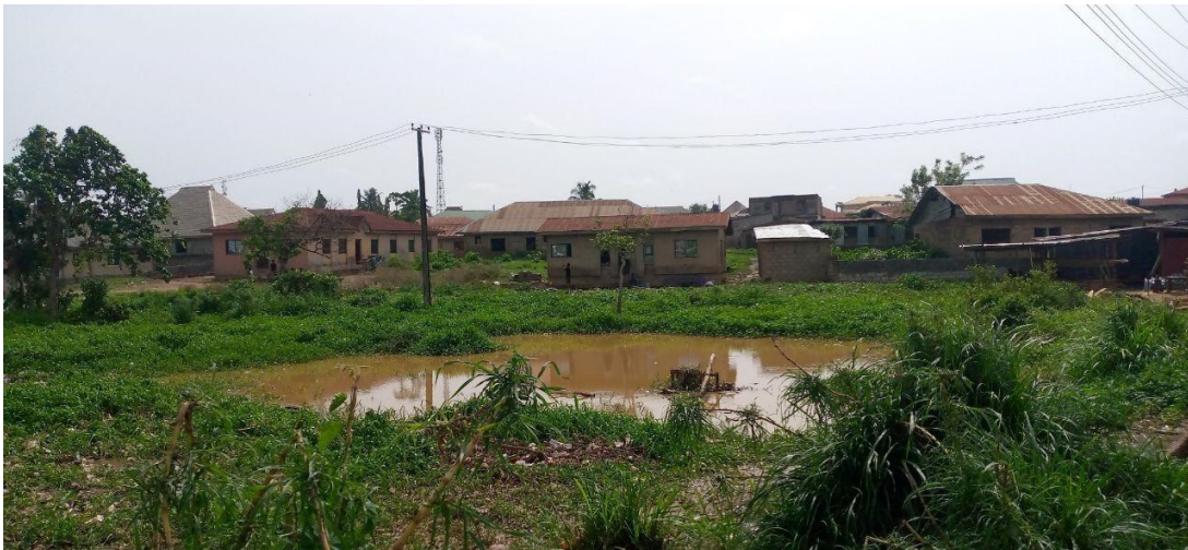
Figure 4.2. Effect of Encroachment on Oil Pipeline in the Ologuneru Area
